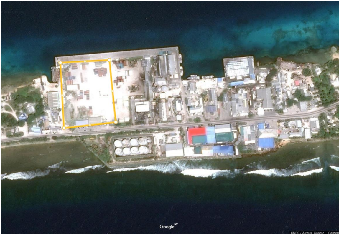
Figure 3: Map showing required land area for batteries on Majuro (5 acres) near the power station
