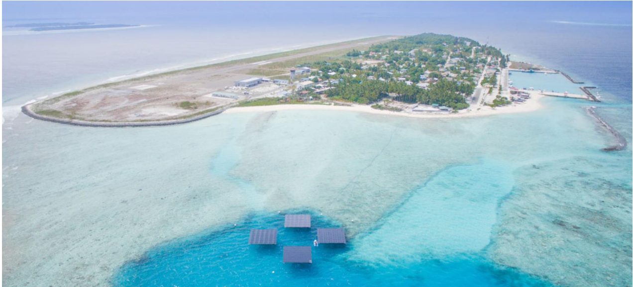
Figure 1.4 - Solar PV - Lagoon floating trial installation in Baa Atoll, Maldives (Source: Swimsol company)
